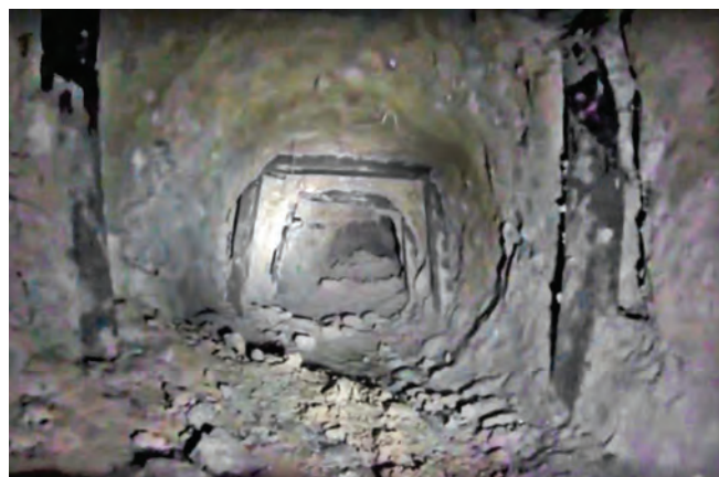
The tunnel was photographed using a remotely controlled camera
